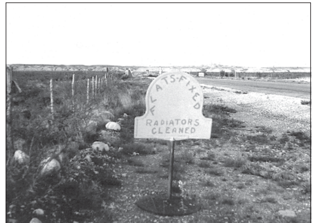
Hope! Flats repaired somewhere ahead. James Reddell.
