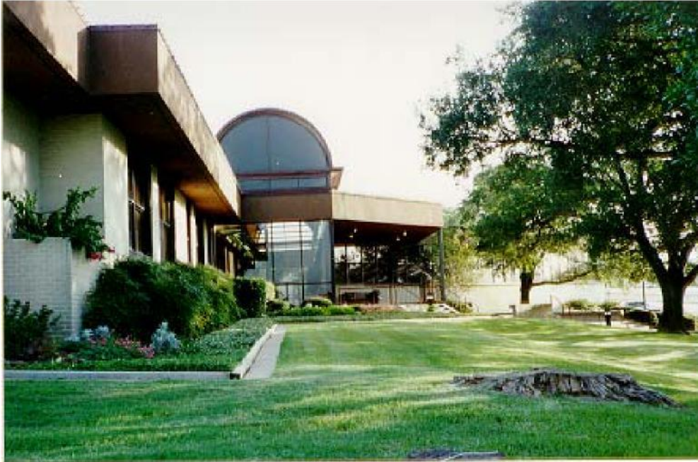
Fig. 33 Exterior view of conference center
