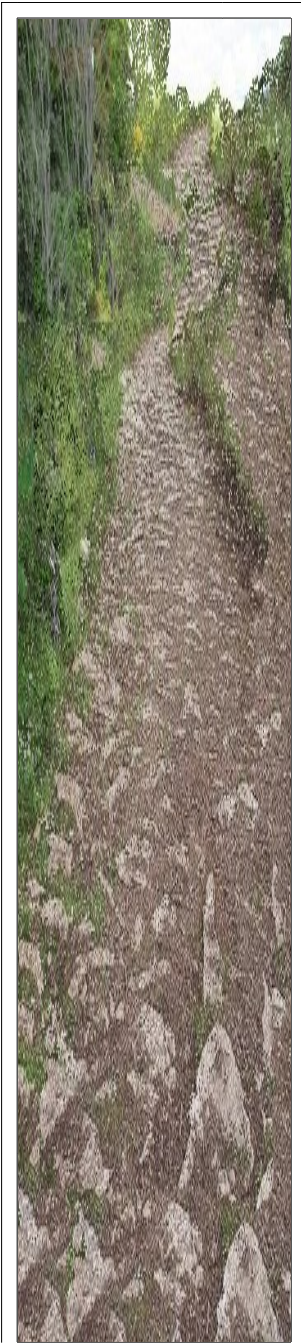
The Romans constructed the Egnatian roadway in the 2nd century B.C. It was a little more than 19 feet wide and paved with stone slabs and layers of sand.
