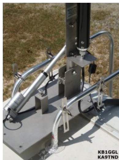
Picture 4 – MT-1 & Automatic Lift & Lay
