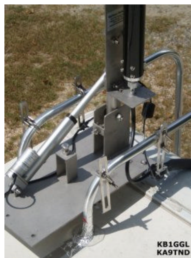
Picture 4 – MT-1 & Automatic Lift & Lay
